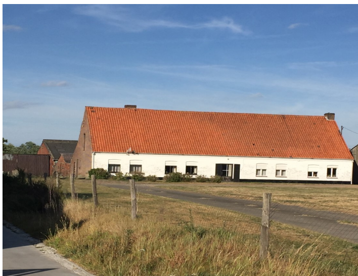
33 Squadron Dispersal HQ Building , Maldegem Association Battlefield Tour Final Stand Day One
